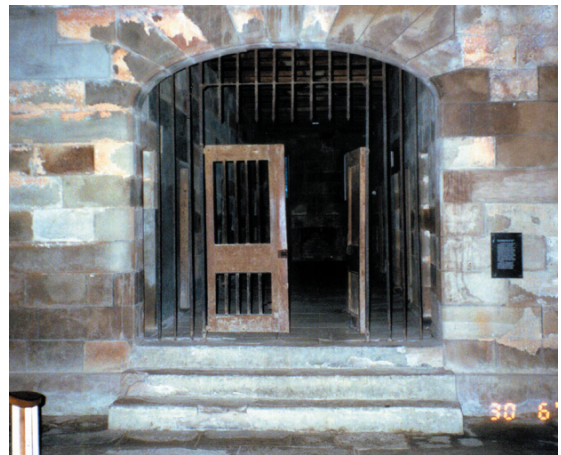
↑ Figure 5.5.2.3 Entrance into A Wing showing steps
