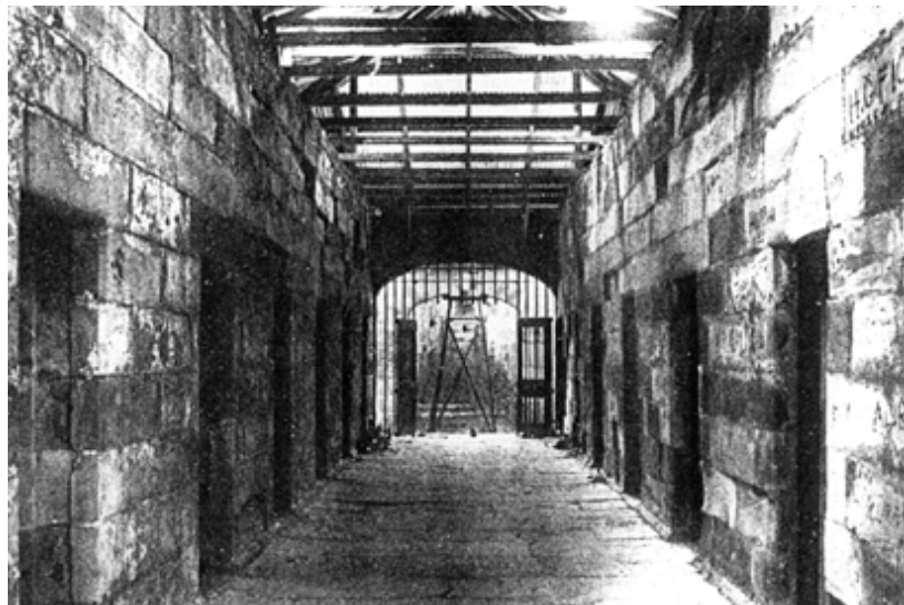
Figure 2.2.2.6 Interior of A Wing roofed and with the iron grill into the Main Hall. Note also the Prison Bell beyond the grill (PAHSMA photo archive 2170)
