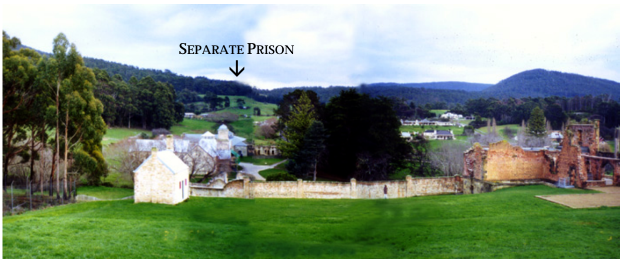
Figure 2.6.14 View towards the Separate Prison from in front of Smith O'Brien's cottage
