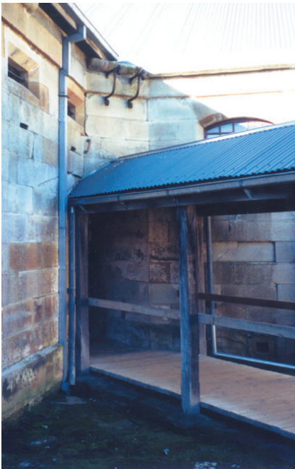
↑ Figure 5.5.2.1 Boardwalk into Central Hall
