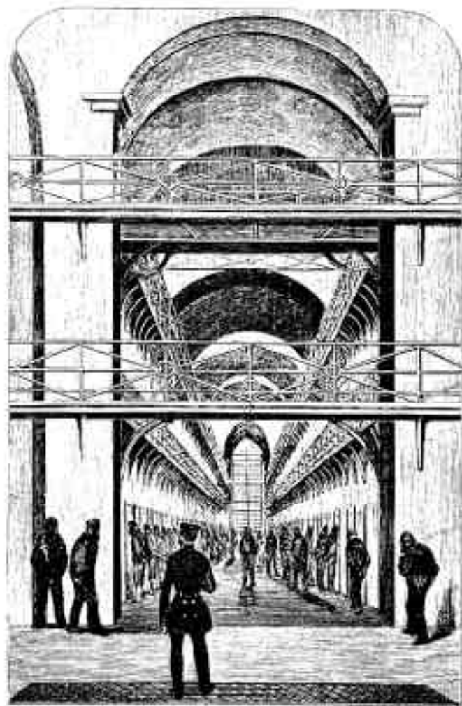
SECTION OF THE PENITENTIARY HOUSE OF CORRECTIONS, WANDSWORTH, WITH THE PRISONERS PUNISHING THE AURAL STAKE.
