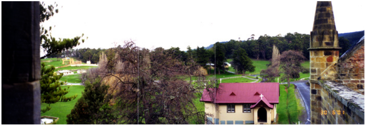
Figure 2.6.4 View towards the Separate Prison from the church tower. Part of it is just visible above the red roof of the chapel
