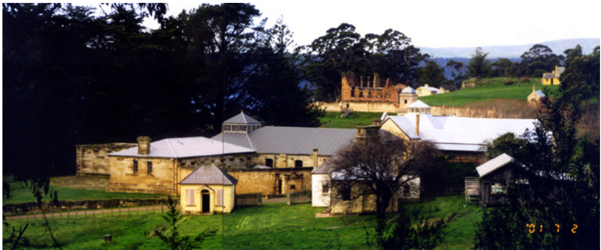
Figure 2.6.12 View towards the Separate Prison from above tramway cuttings (c.f. historical views in Figures 2.4.2.1 and 2.4.2.2)
