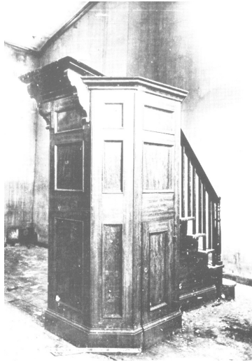
Figure 5.8.11 The original Pulpit in the Chapel of the Separate Prison (PAHSMA Photograph Archive 1275)
