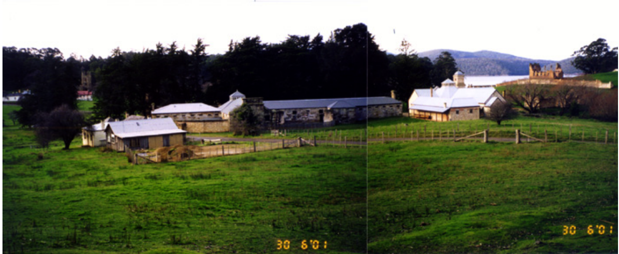
Figure 2.6.13 View towards the Separate Prison from across "The Farm"
