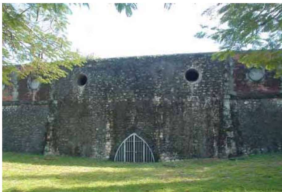
Water Reservoir, Nouméa, New Caledonia.
