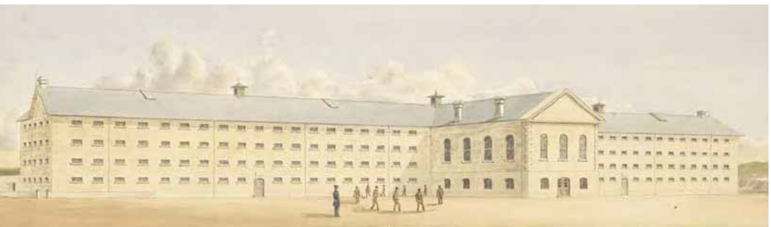
Main Cell Block of Fremantle Prison in 1859 showing convicts and a guard.
