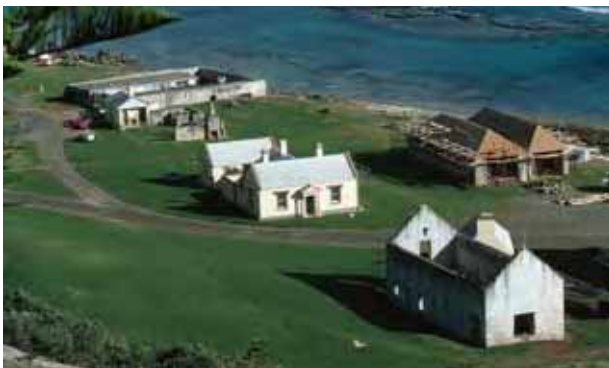
From left to right; Prison Compound, Royal Engineer's Office and Stables, Double Boatshed and Crankmill.
