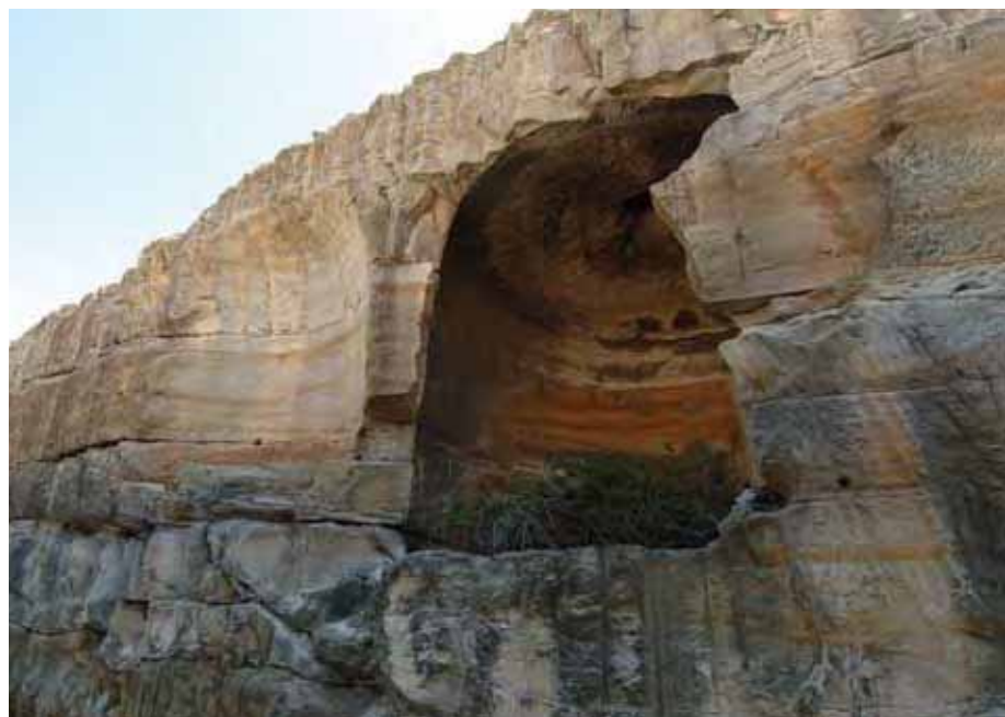
Sandstone grain silo hand cut by convicts, exposed on the edge of the cliff.
