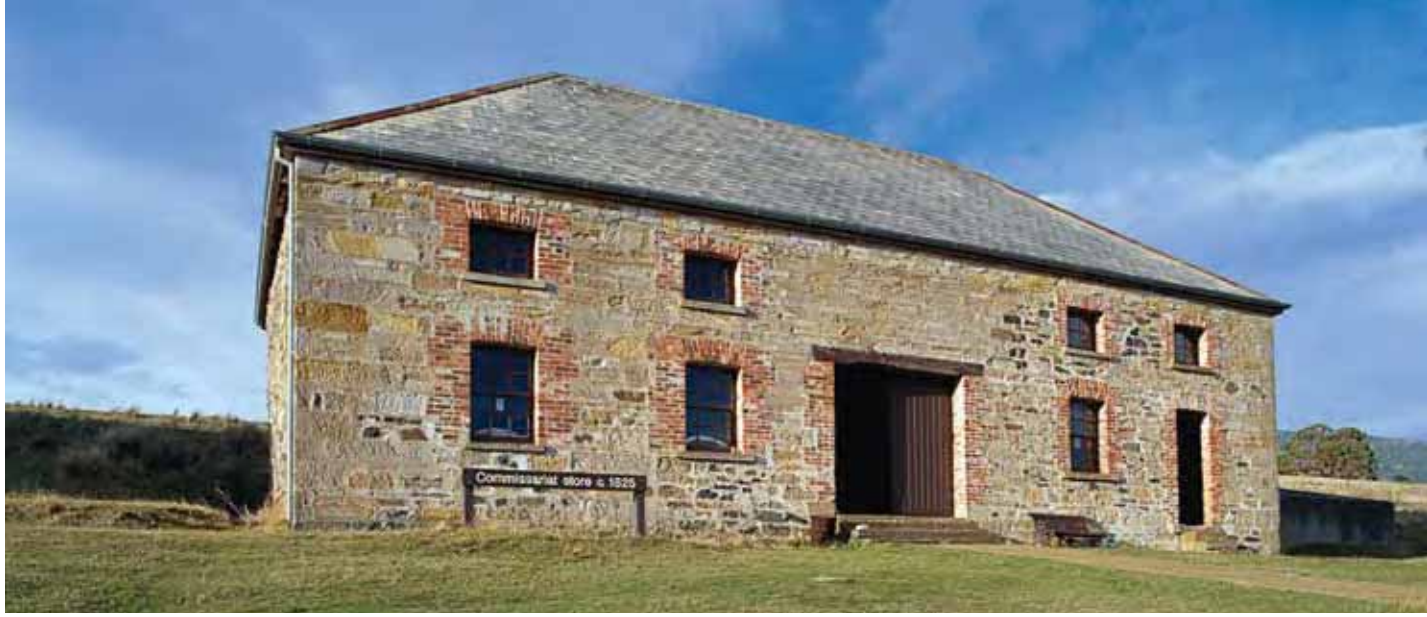
c.1825 Commissariat Store at Darlington Probation Station.
