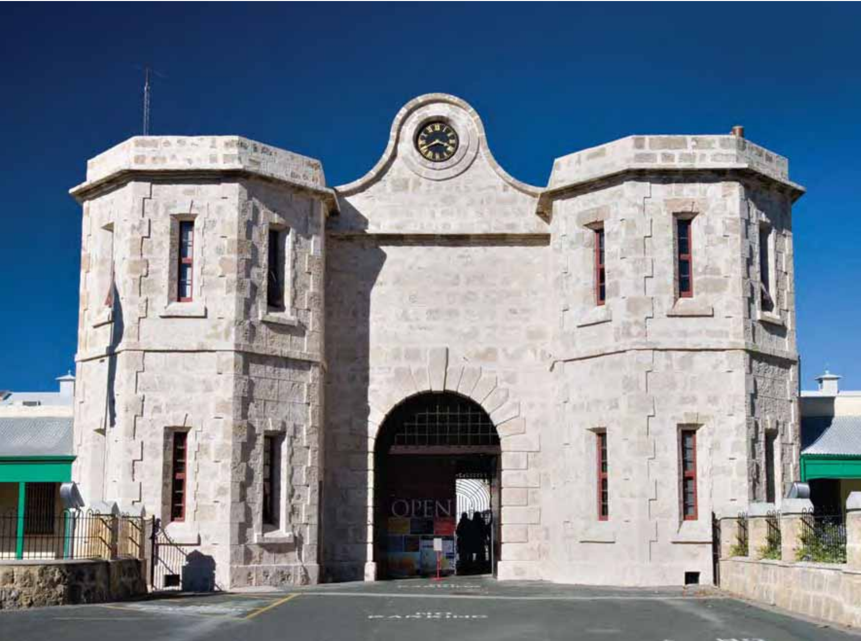
Fortified Gatehouse entrance to the prison.
