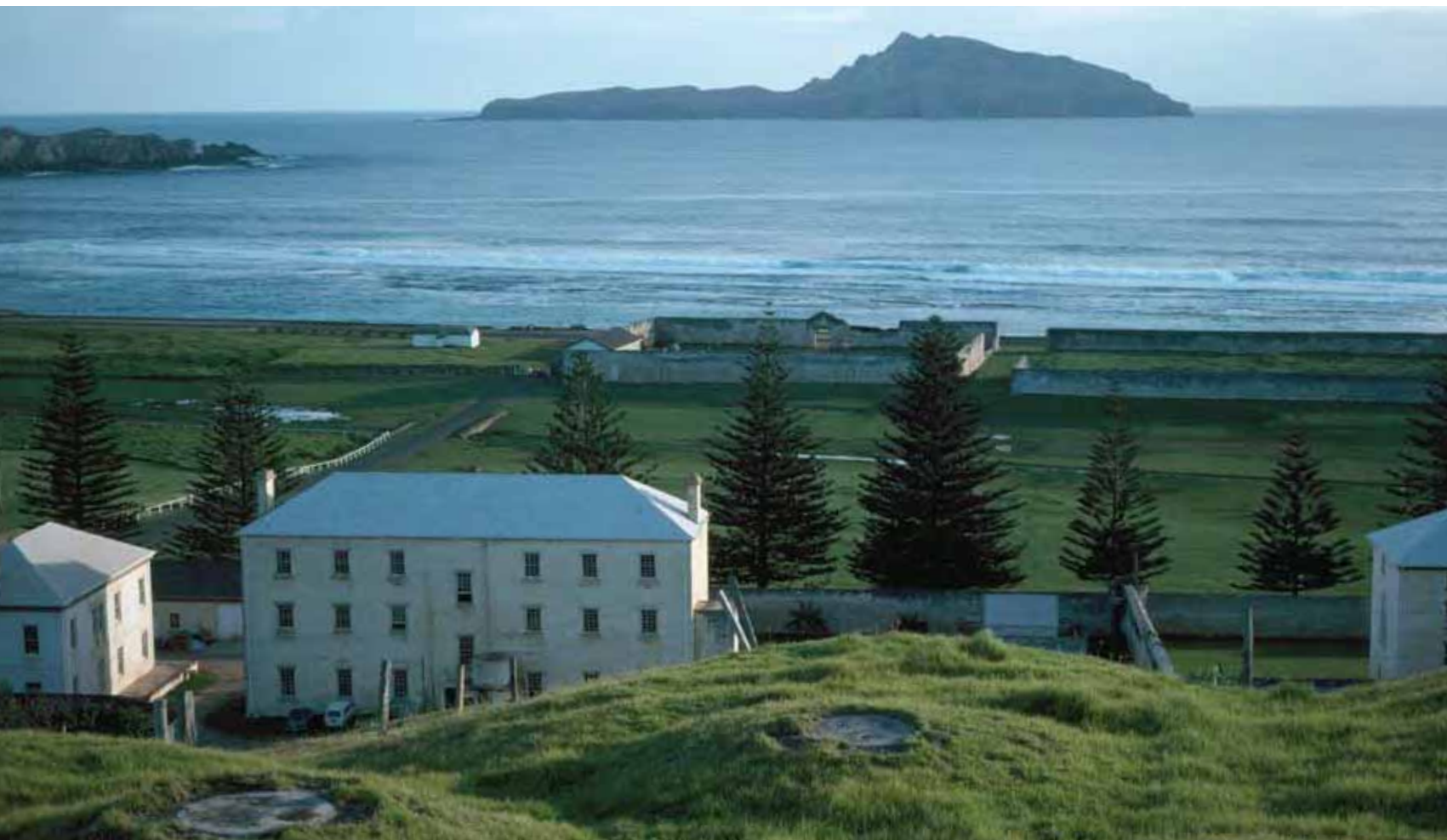
The Commissariat Store and New Military Barracks in foreground with Convict Barracks and Prisoners' Compound with New Gaol in background.
