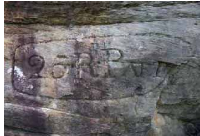
The convicts of the No. 25 Road Party gang marked their presence in the rock wall. Graffiti were often used as a form of resistance against penal servitude, and sometimes as a mark of pride in their work.
