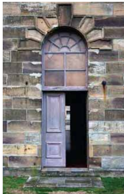
An entrance to the Mess Hall, Cockatoo Island.
