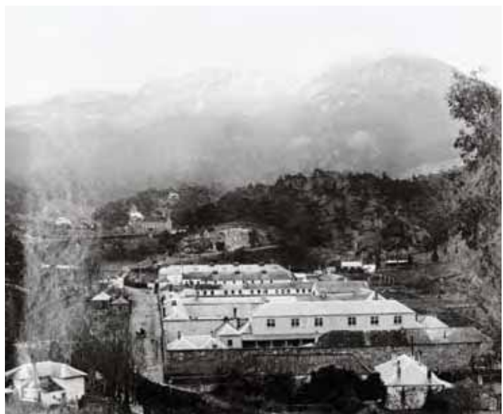
The original five yards with the Nursery and Matron's Cottage in the foreground.
