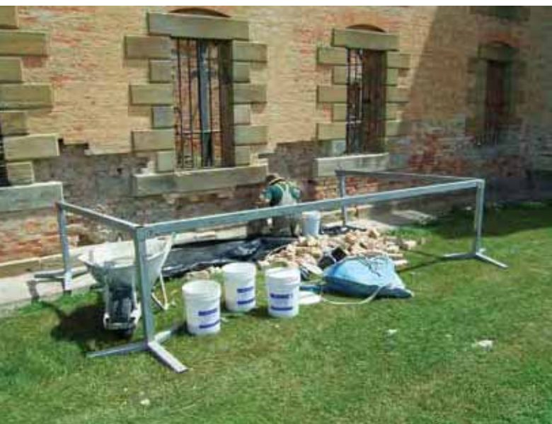
Conservation work at Port Arthur.
