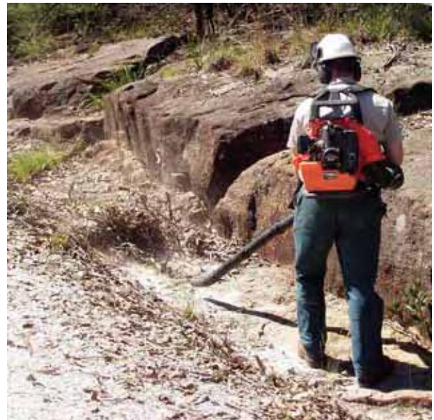
Ongoing maintenance works to remove vegetation growth at Old Great North Road.
