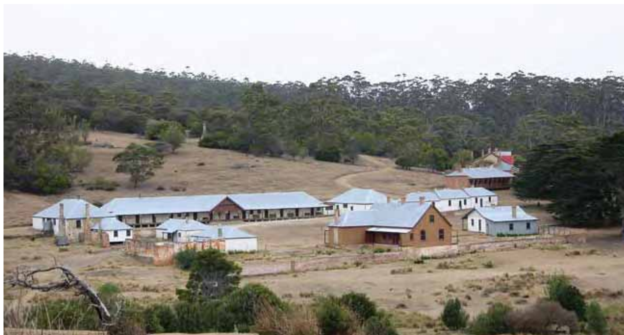
'[T]here were few stations that could lay claim to any approximation to the superior system observable in the Darlington Probation Station' Acting Governor LaTrobe 1846. 77
