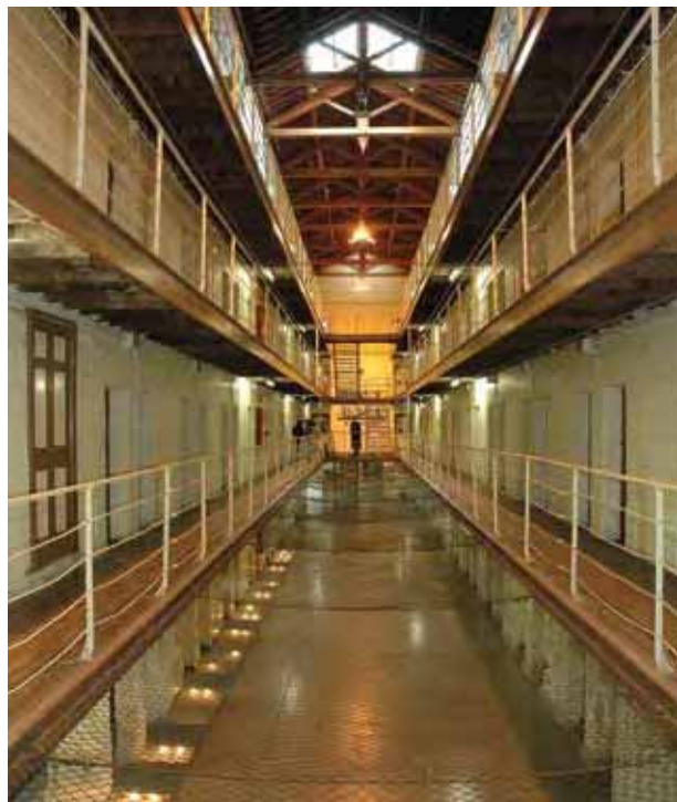
Interior of one wing showing elements of Pentonville design with front facing cells along galleried walkways.
