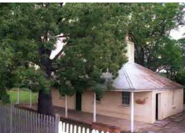
The Governor's Dairy built by ex-convict George Salter on land granted in 1796. The building was later extended by Governor Macquarie.
