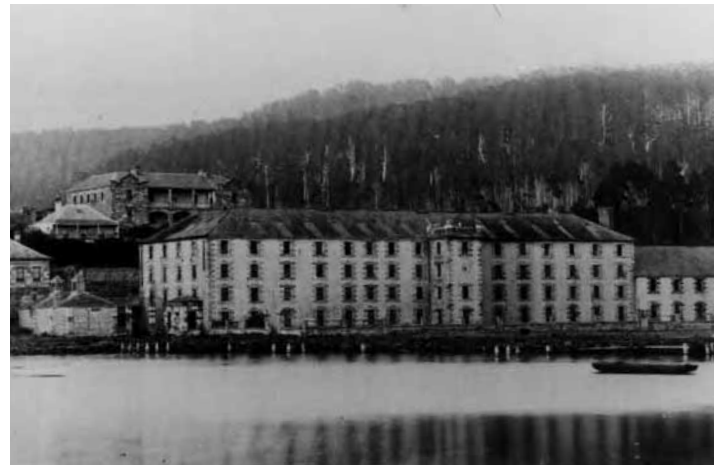
Historical photograph of the four-storey Penitentiary.
