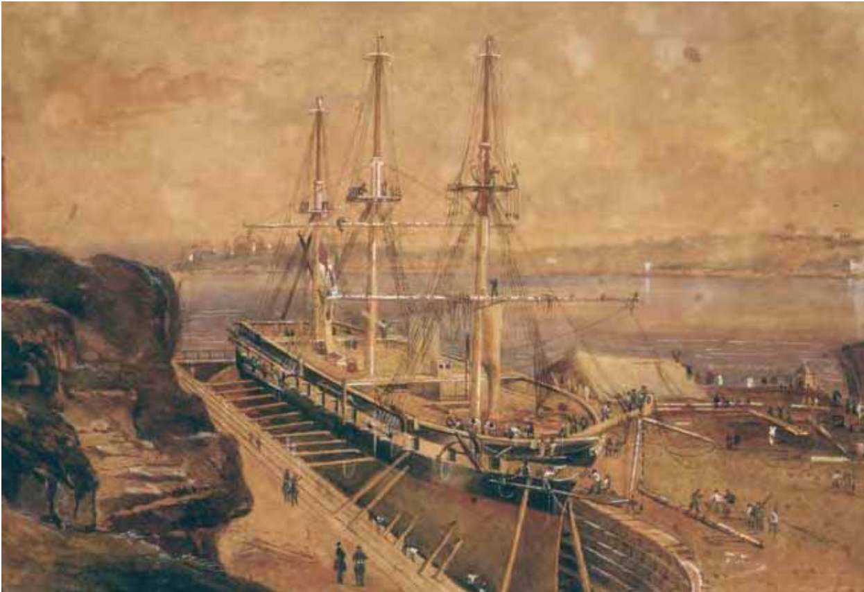
HMS Galatea in Fitzroy Dock, Cockatoo Island. Convicts significantly contributed to the construction of the dock enhancing Britain's naval influence in the Pacific.
